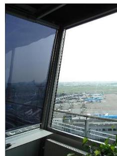
Sunblinds at a traffic-tower.
